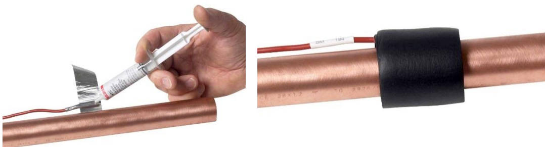
Figure 2 - Apply sensors with heat transfer compound, Aluminium and insulation
